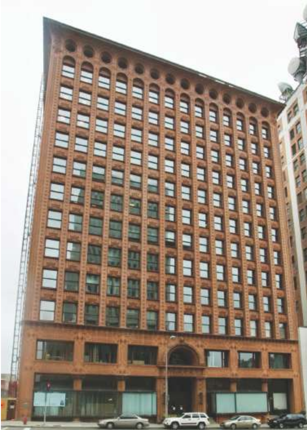
Figure 3: Louis Sullivan, Guaranty Trust Office Building , Buffalo, New York, 1894–96, steel, terracotta and glass
