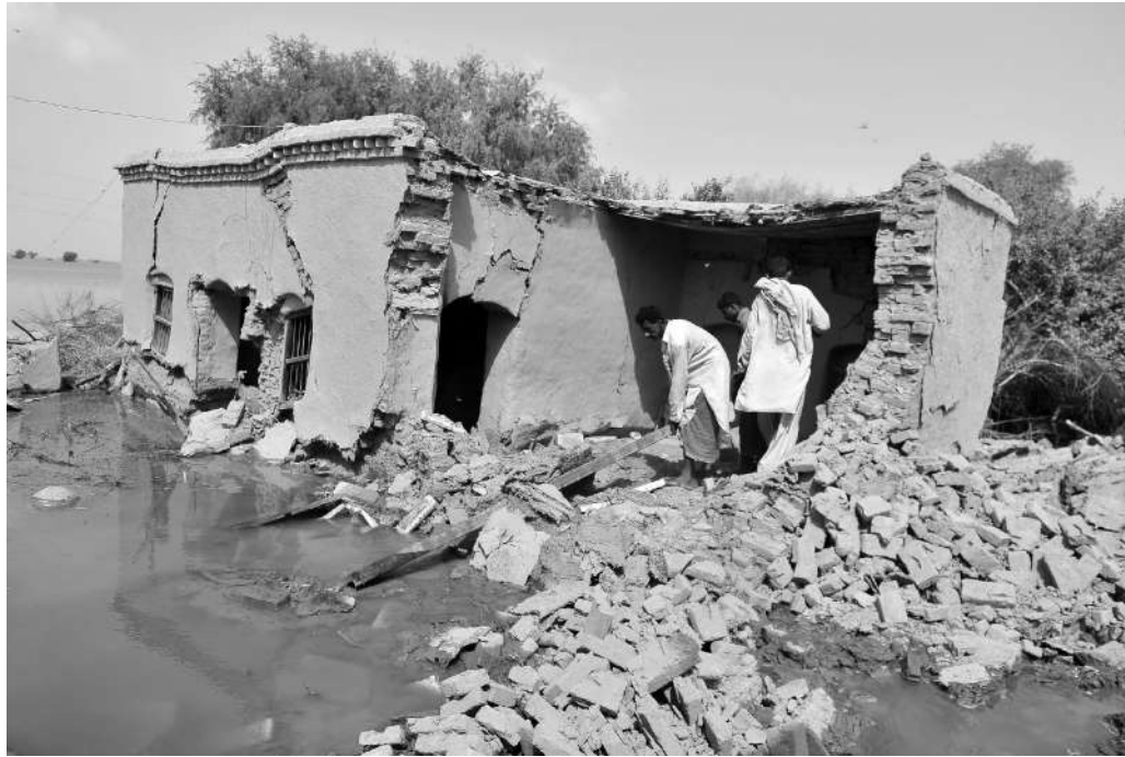
Earthquake Damage in Pakistan (2010)
